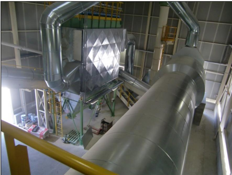
Figure 25: Drying system TRH for screened limestone
